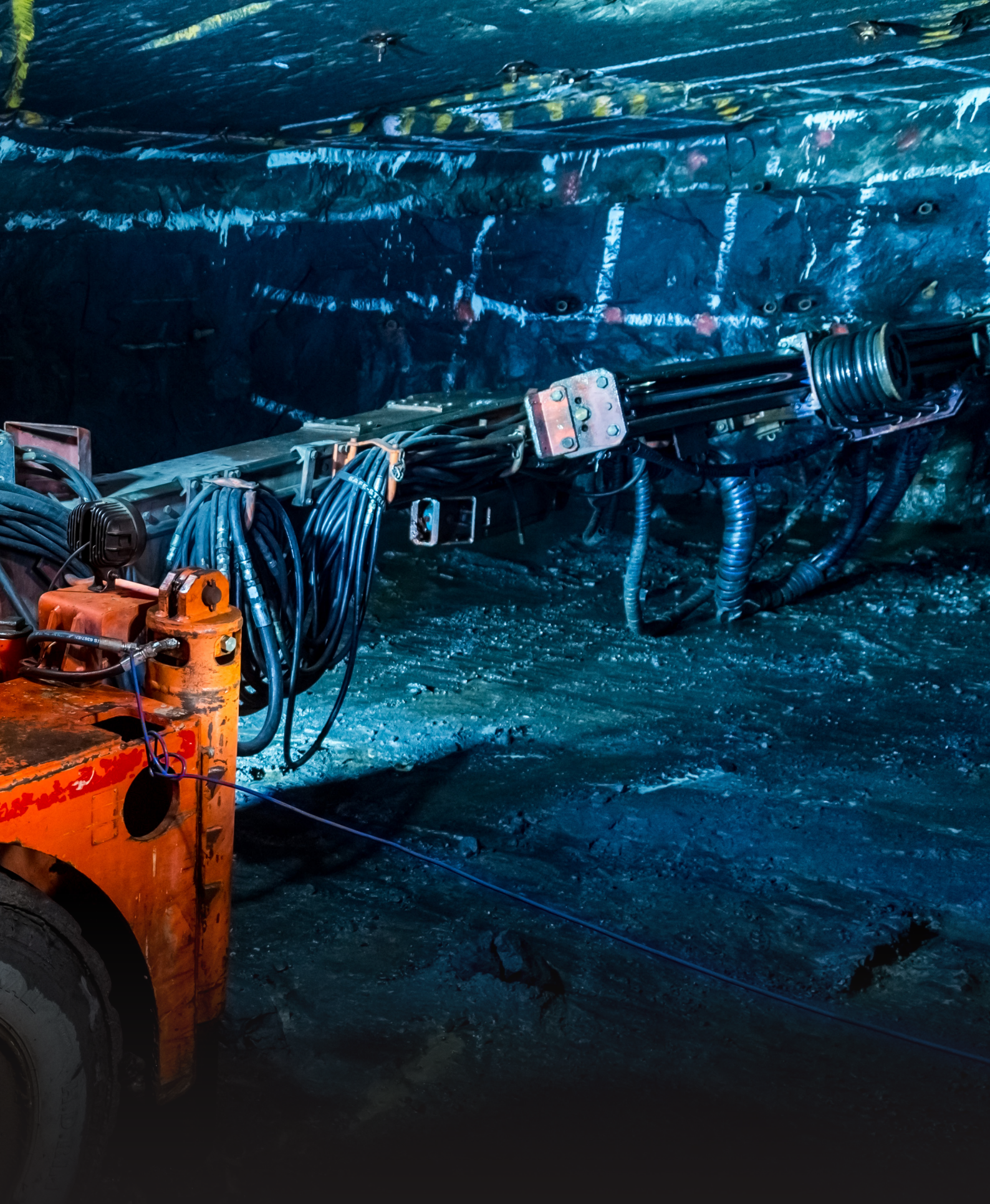
Dwarsrivier Chrome Mine underground face drilling
